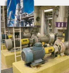
Easy-Laser® is used to align pumps and motors for all types of installations in a variety of industries. Correctly set-up and aligned machines are necessary to reduce energy consumption and achieve optimum service life.
